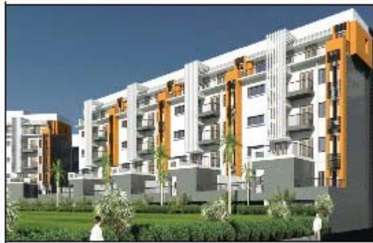
Iris Court, Mahindra Integrated Township Ltd, Maraimalai Nagar, Chennai
