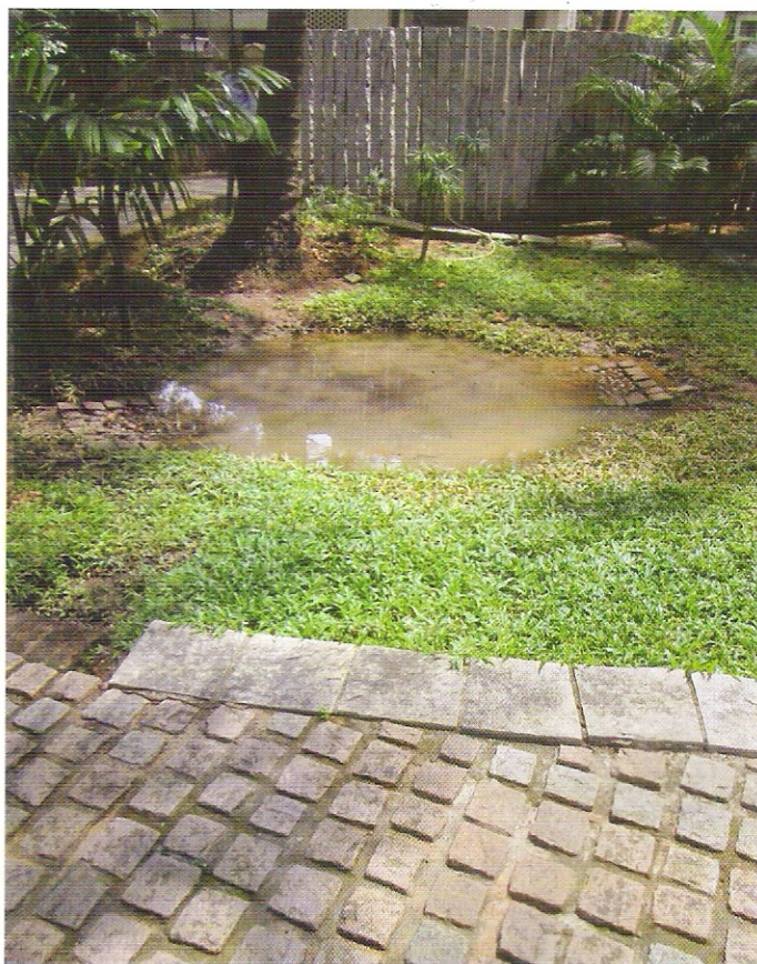
a swale that is filled during the monsoon helps keep the rest of the landscape from flooding; Residential development, Chennai.
