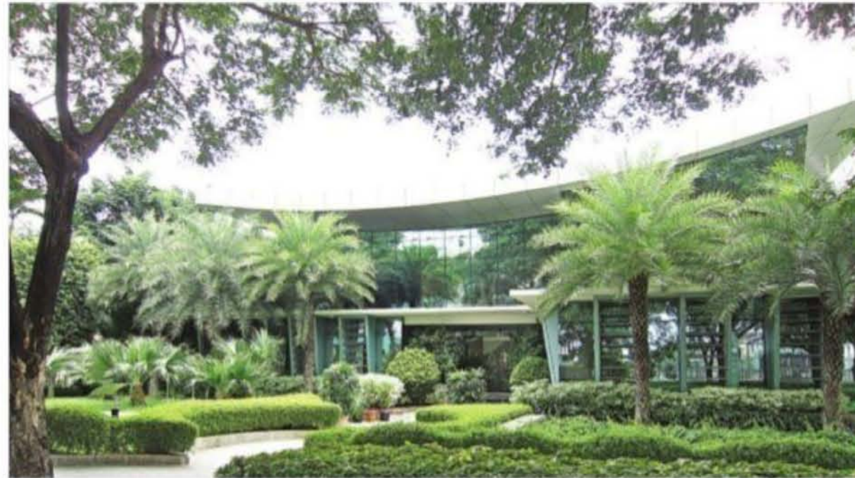
Glazed walls add to the beauty of the facade
